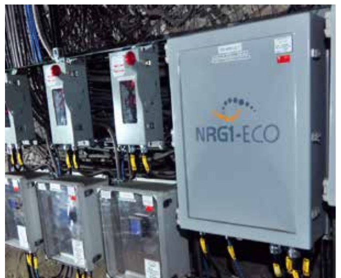
Figure 104: BESTECH's NRG1-Eco system to minimize electricity consumption costs associated with auxiliary mine ventilation systems. Source: http://www.bestech.com/Downloads/ProductSheets/BESTECH_NRG1-ECO.pdf
