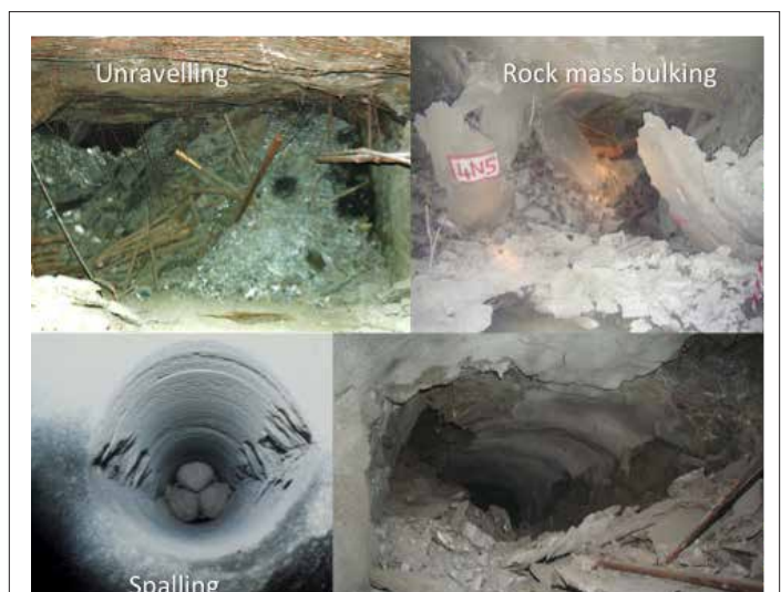
Figure 11: Examples of excavation instabilities in stressed rock
