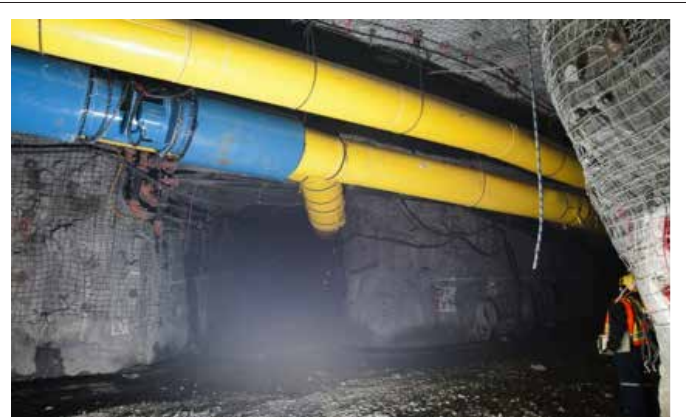
Figure 111: The yellow sections of the auxiliary ventilation system pictured above are novel low friction plastic ducting segments that are supplied by Gplus Industrial Plastics Inc.. Source: www.plastiquesgplus.com/en/ventilation
